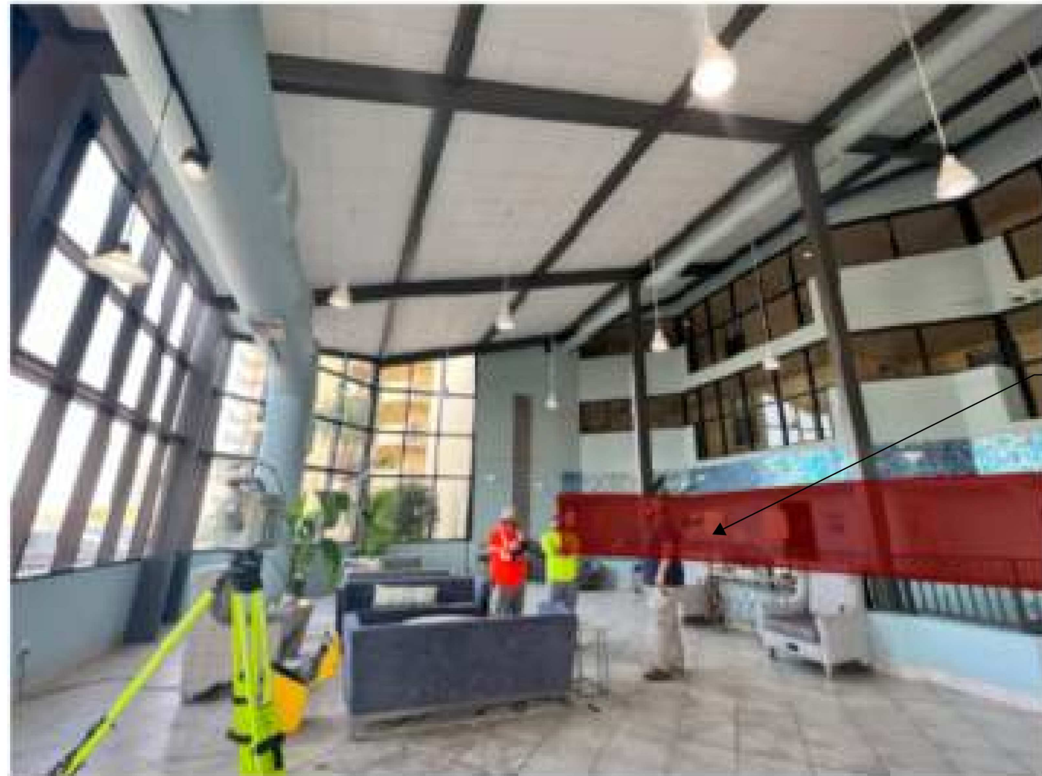
INSTALL CONSTRUCTION BARRIER AT UPPER LEVEL CONSTRUCTION AREA
