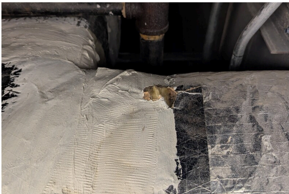
Photo 6: HA05: White Duct Mastic
