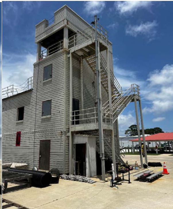
Southwest elevation view
